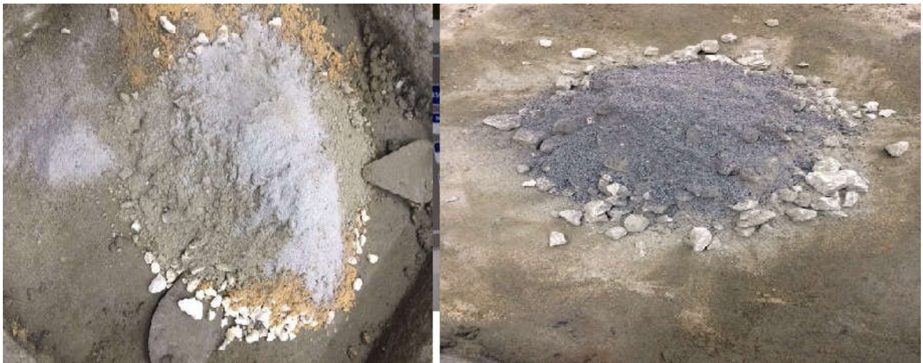
Figure 1. Preparing the concrete mix components by hand
